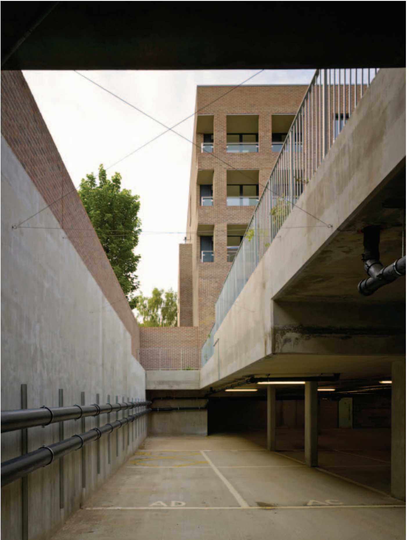
Block from basement car park
